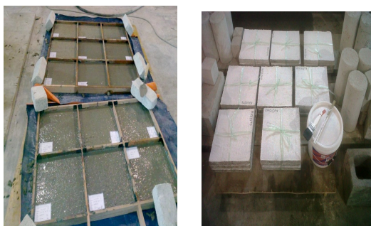
(a) Casting of slabs (b) Surface whitewash
